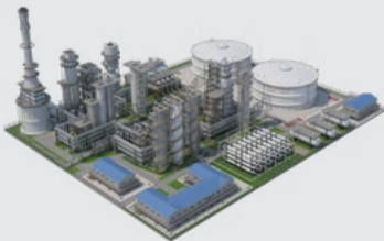
Central Power Plant
